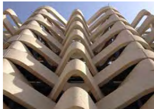
Cooling Tower, Doha
