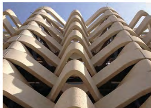
Cooling Tower, Doha
